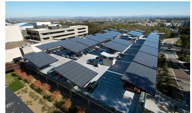
Microgrid CHP and solar generation, photos courtesy of LBNL and UC San Diego
