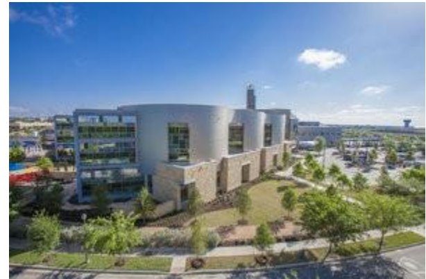
Dell Children's Medical Center, photo courtesy of Seton / Ascension
