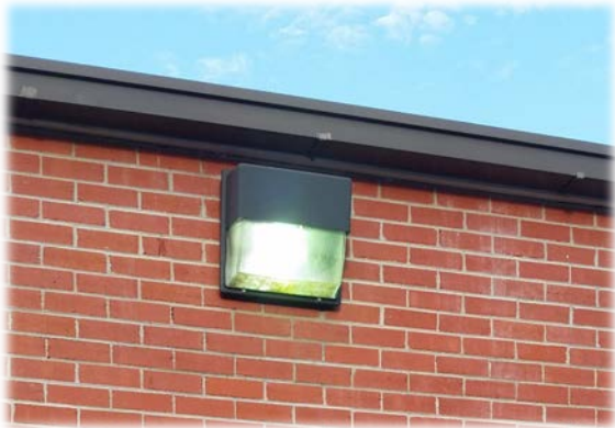
Malfunctioning Photocells
