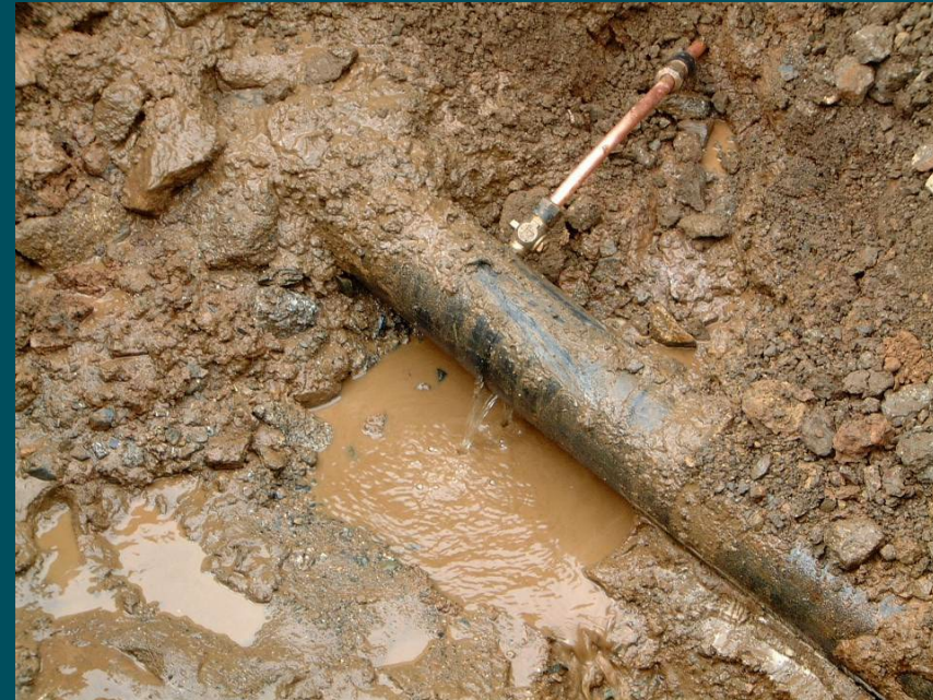
Low-Pressure Leak
